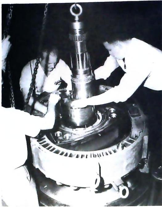
Figure 12. - RC1-1920 engine, assembly of power section.
